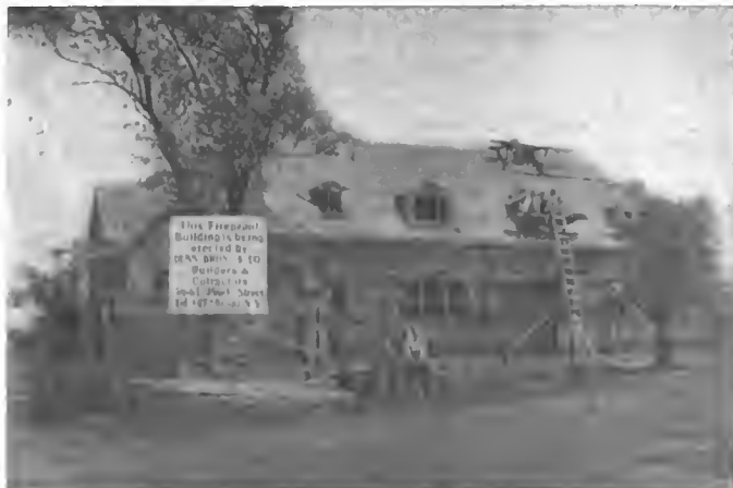
Hollow Tile Garage In Process of Construction
